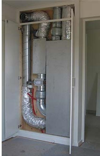
*Fig. 2.4.1: Illustration of a heat recovery unit placed in connection to the ventilation system in a closet. This solution makes the maintenance easier.*
