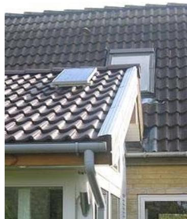
*Fig. 2.9.1: Small ventilation unit for sunspaces which is operated by help of a small PV-plant, which produces the needed electricity for operation of the fan. A operation the fan. A ventilation rate up to 400 m<sup>3</sup>/h is possible. FK: The PV module is about ¼ m<sup>2</sup>, so it generates about 25Wpeak, which is far too little to drive the heat pump.*
