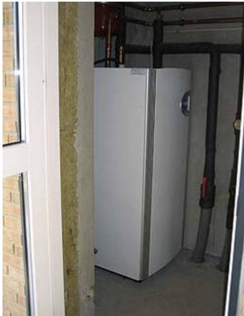
*Fig. 2.8.1: Heat pump producing heat for 8 apartments using heat from the ground.*
