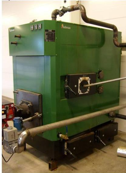
Figure 7. Connection of syngas burner to the fuel oil boiler.
