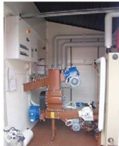
Figure 4. Bioboiler and fuel intake are located in the same container.
